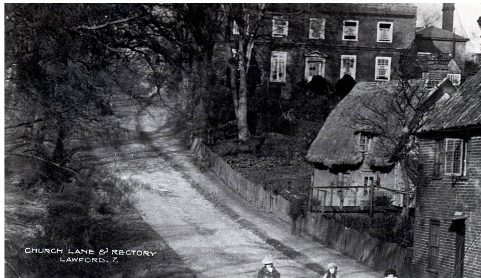
Figure 5 Photo of Church Lane, Rectory
